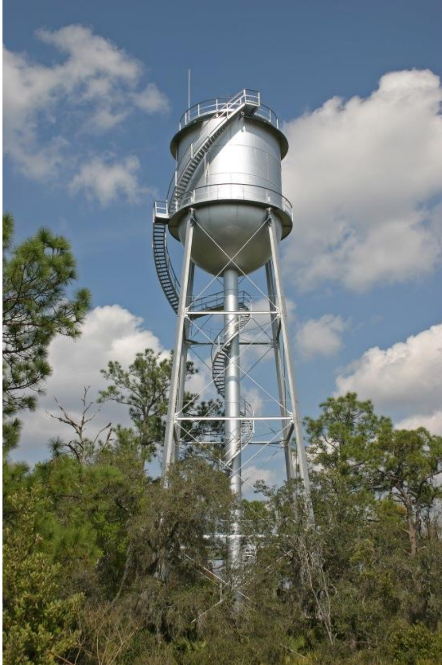
Archbold’s water tower pumps potable water up from the Upper Floridan aquifer and can store 75,000 gallons in its tank. Photo credit: Archbold Biological Station.
